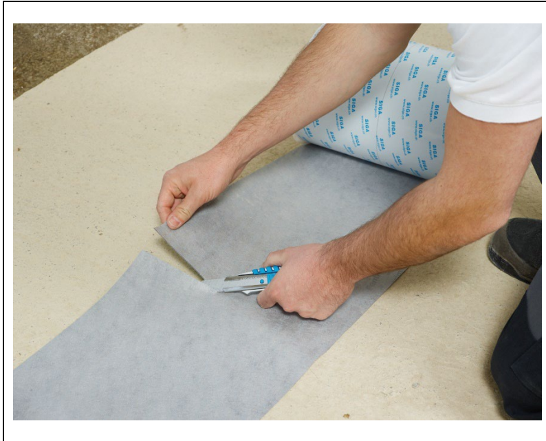
Figure 2 Cutting tape to length
