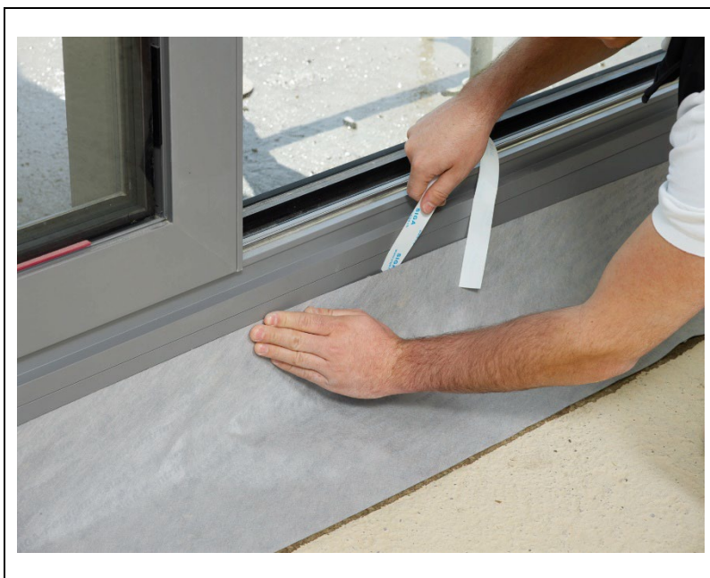
Figure 4 Removal of release film
