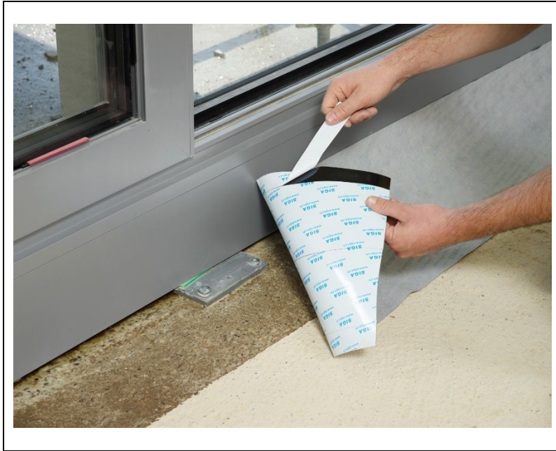
Figure 3 Starting removal of release film
