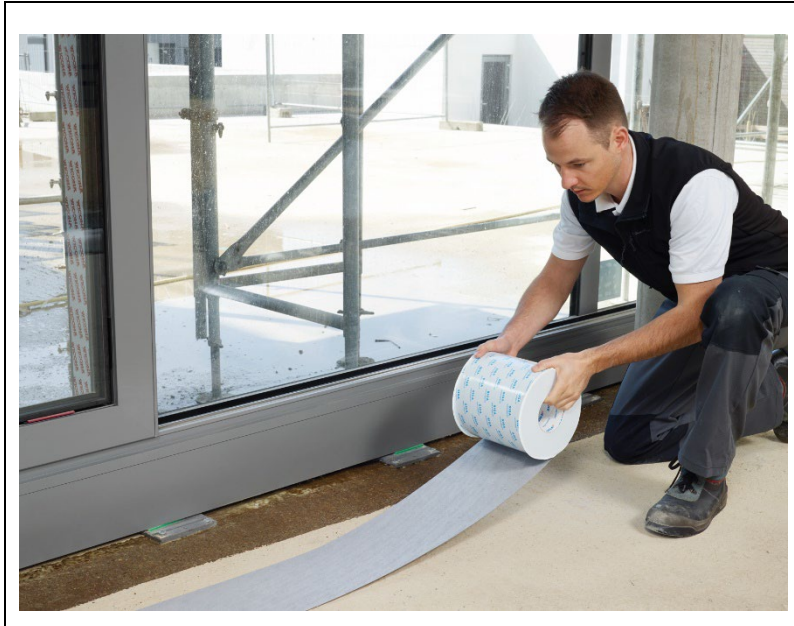
Figure 1 Laying out tape
