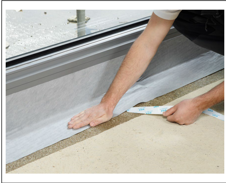
Figure 5 Removal of remaining release films, applied tension free
