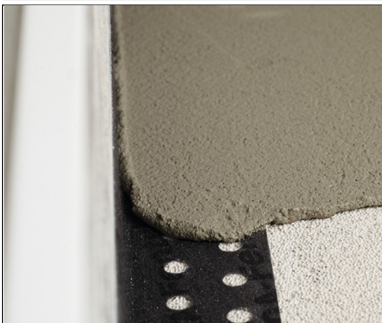
Figure 6 Application of plaster
