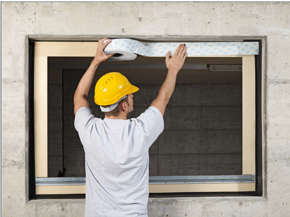
Figure 5 Installing tape at top of frame
