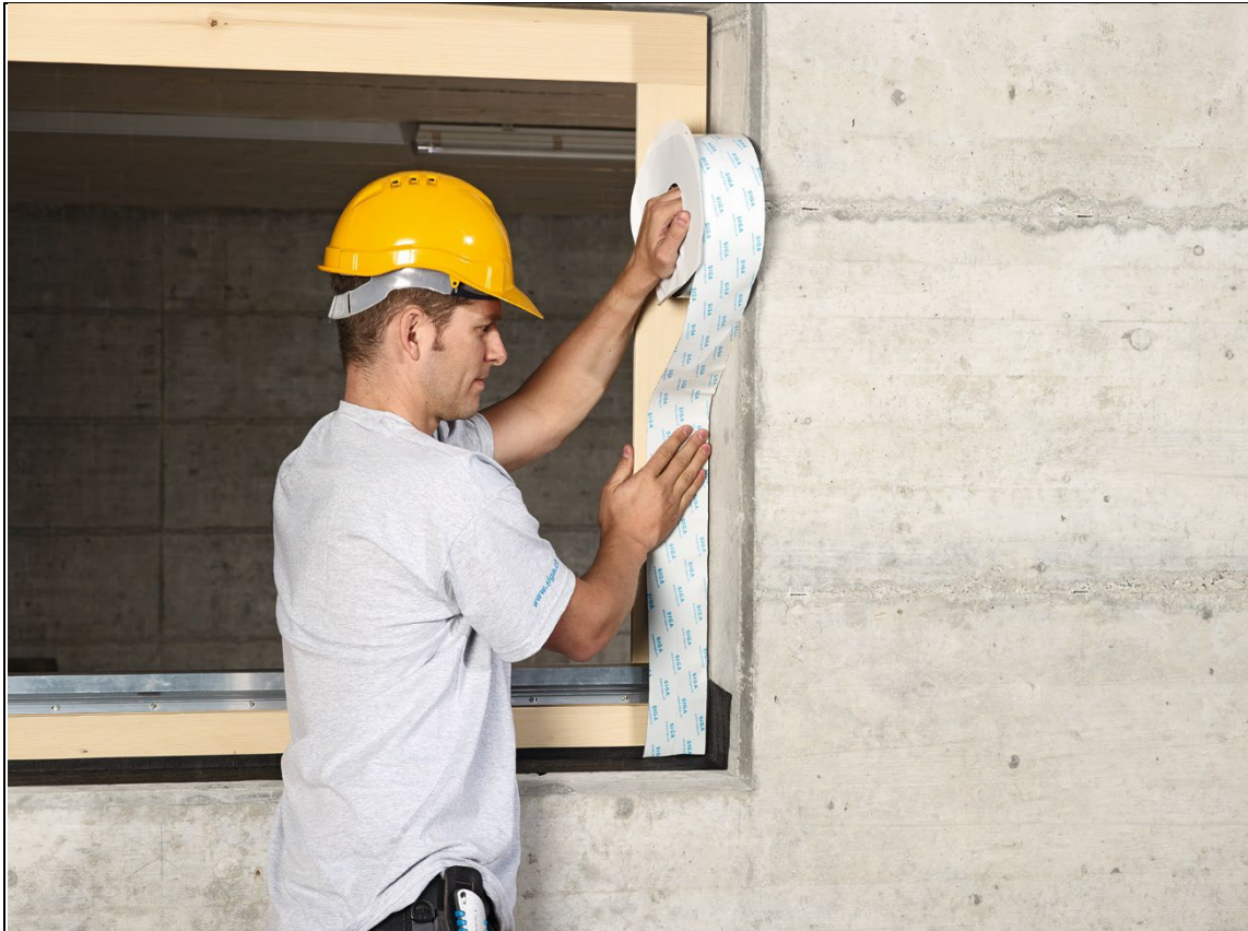
Figure 4 Installing tape vertically
