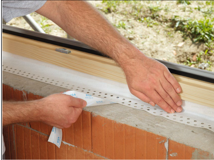
Figure 2 Removal of release film
