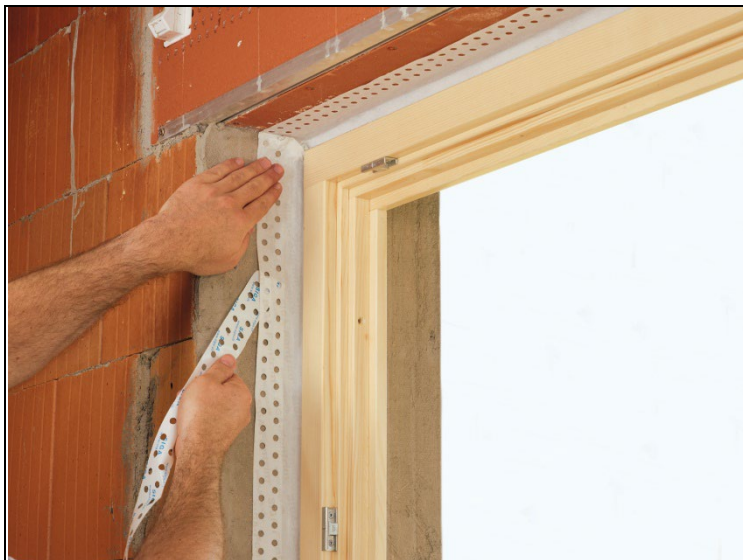
Figure 1 Internal window – corner detail
